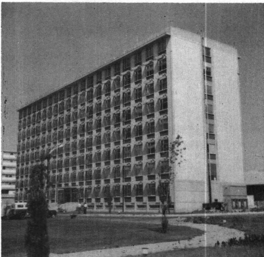
Fig. 1 - The new INMG headquarters
